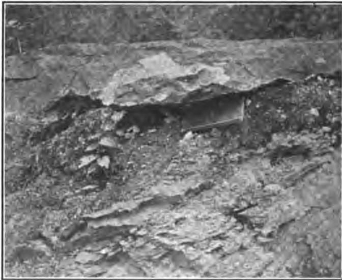
FIG. 978. — Detail of contact of nearly horizontal Potsdam sandstone upon somewhat contorted layers of Grenville quartzite, dipping from 20^{\circ} to 36^{\circ} , looking west. Taken at a distance of 4 feet, the notebook on the contact. One mile southeast of Redwood, Jefferson Co., New York. (H. N. Eaton, photo, 1908. Courtesy New York State Museum, John M. Clarke, Director.)
